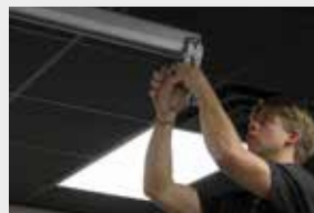
How to Add or Remove a Solo-Step Trolley
